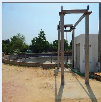
Treatment Plant, Kanpur
